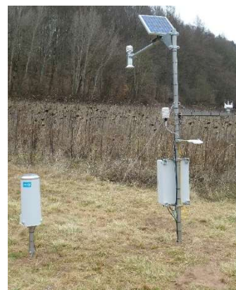
Weather station with snow height sensor and net radiometer, as well as further standard weather monitoring sensors
